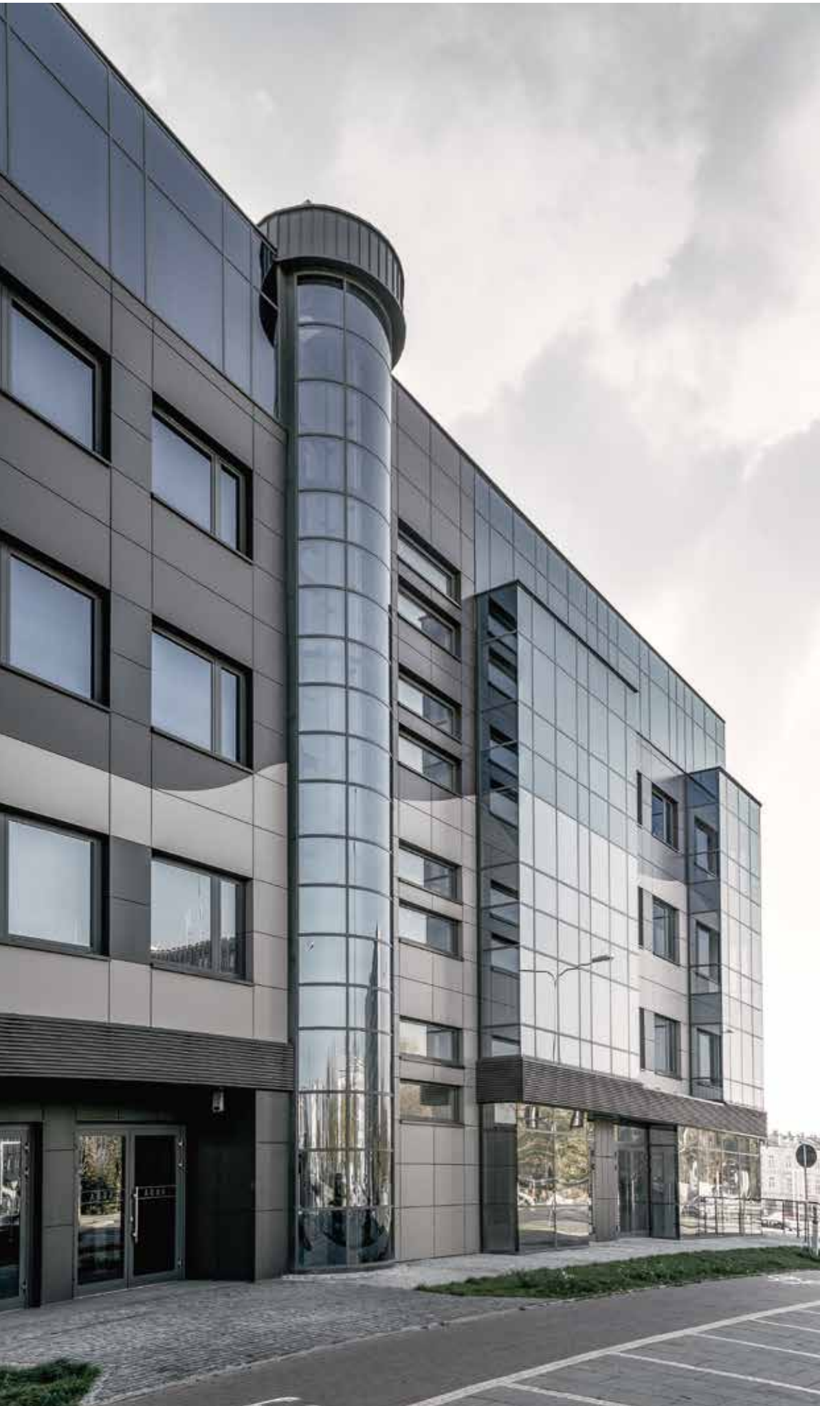
/ Kielce Aqua Office Building Laminam Collection Nero Collection Tortora <
